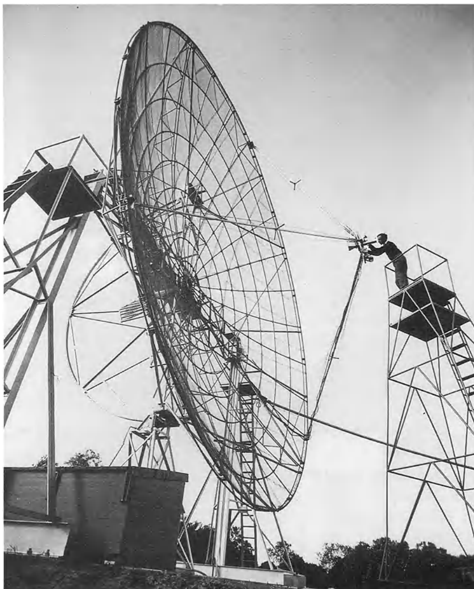
Fig. 5. The 36 ft diameter dish used by Kerr and collaborators for most of their 21 cm hydrogen line work in the 1950's. Working at the focus is Brian Robinson (ca 1953).
